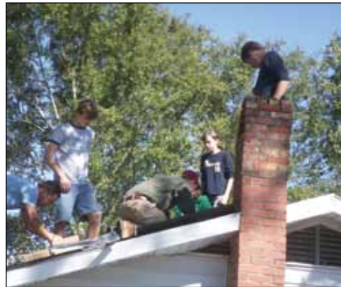
EWB members (left) working on roof damaged by tornado in 2007.
