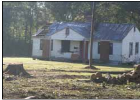
One of the homes damaged in the October 2007 tornado (left).
